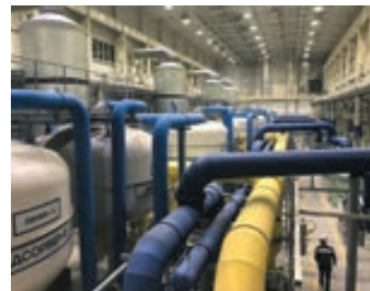
First project: the oxygen generator which has been delivered
