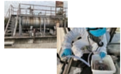
detoxification work for the odorant equipment of LP gas
