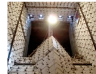
Example installation of irregular refractory bricks
