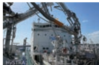
Steel pipe-type loading arm for liquefied hydrogen in connection with a tanker
