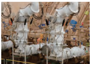
Emergency Release System (ERS unit)
